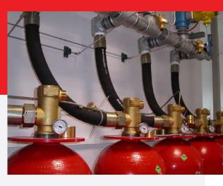
Novec 1230 fire suppression system uses an inert carbon-based chemical that powerfully fights fire yet is safe for property, people, and environment. It looks like water but does not cause the damage normally associated with water because it contains no moisture. The result is lower repair bills and less impact on business.
